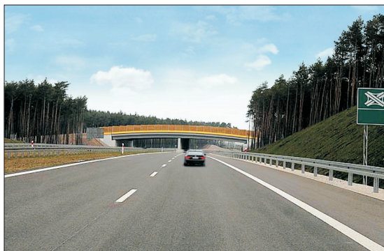
Fig. 4. Expressway S8 – exposed aggregate finish
